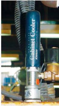
Six years later, this manufacturer contacted EXAIR for another application. They mentioned the old EXAIR Cabinet Cooler system still on the motor drive panel, cranking out cold air. No maintenance had been performed on the Cabinet Cooler System in that time (as none was necessary) even though the environment was quite dirty. It was still working perfectly!
